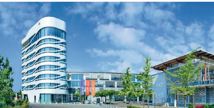
The Innovation & Gründerzentrum Biotechnologie (IZB) in Martinsried near Munich, home of a number of biotech companies (© IZB)
