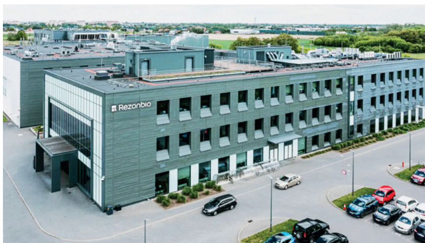
Rezon Bio's FDA certified Gdańsk facility
